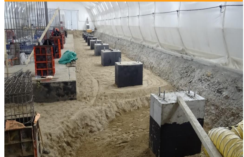
Autoclave and POX building foundations
