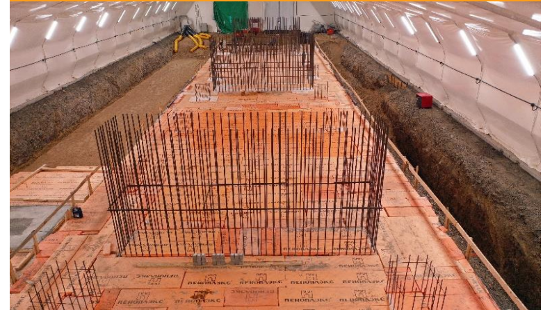
Autoclave foundation inside preservation hangar
